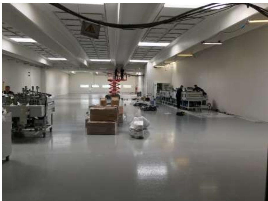
Pic. 1: New plating equipment under installation
